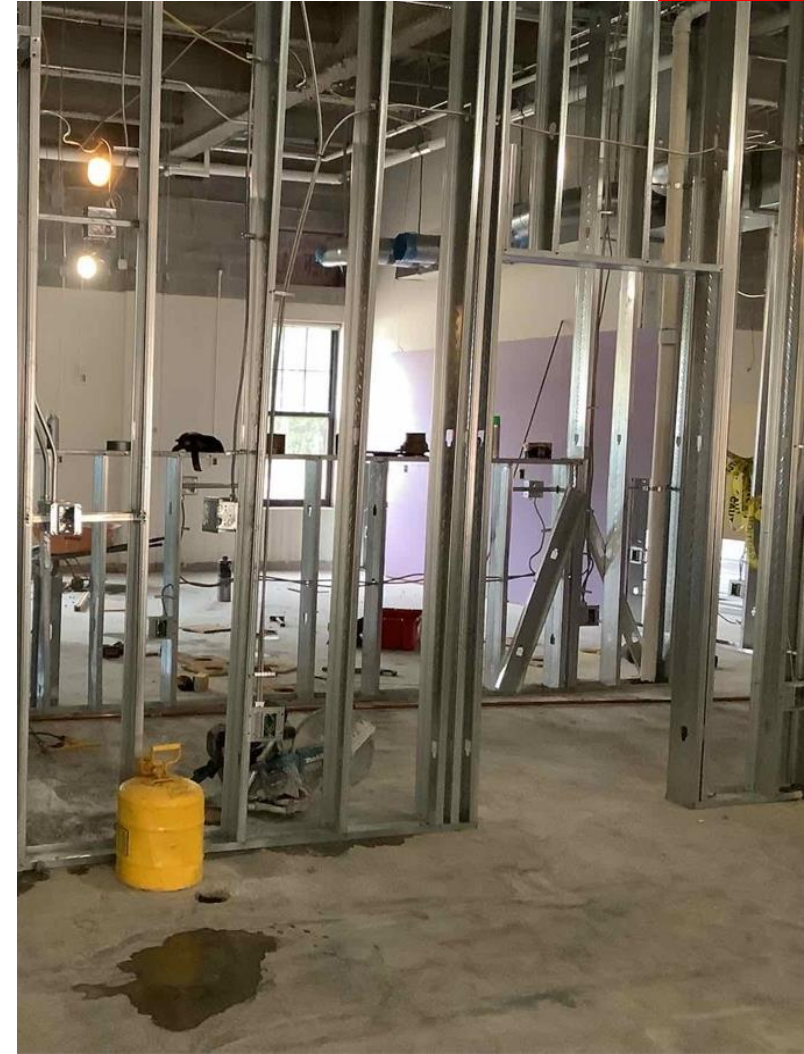
Electrical rough-in at Area D
