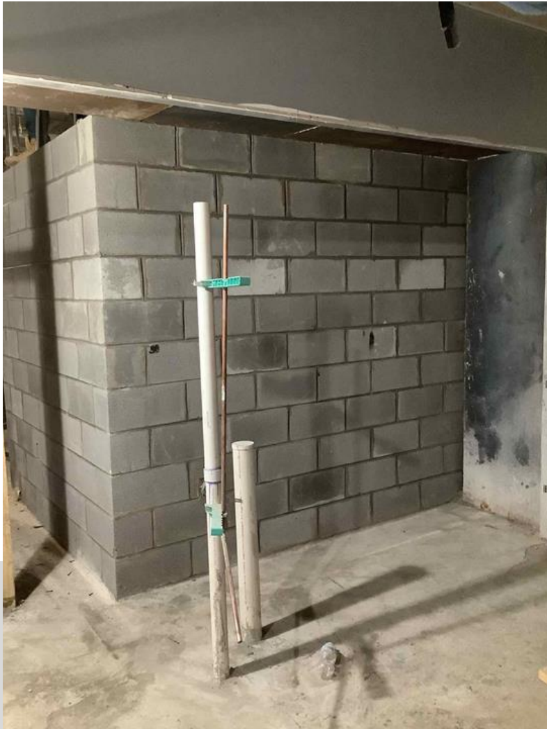
CMU at new elevator shaft
